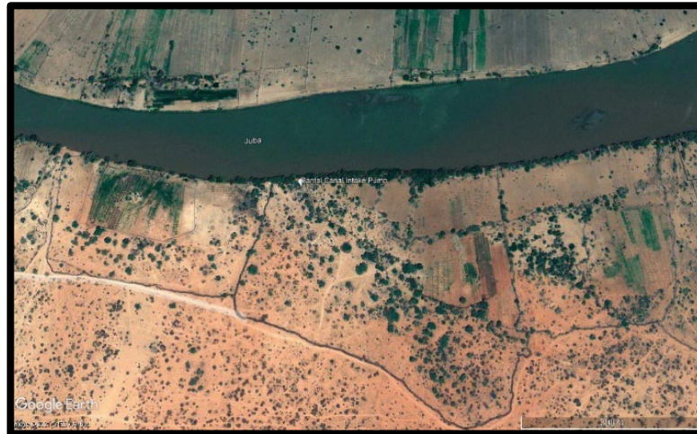
Figure 1: Bantal Canal Intake Pump: Google Earth imagery, September 2012
