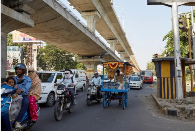
Elevated railway in Nagpur. Source: KfW photo archive, photographer: Davin Meckel
