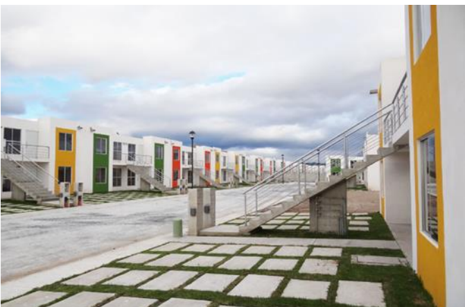
On average, an EcoCasa house uses 20 % less energy than a comparable standard house. Source: KfW photo archive / Klaus Veigel
