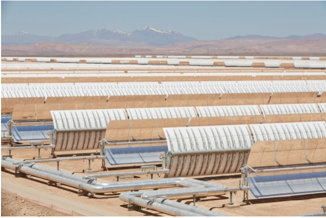
Solar field of NOORo I. Source: KfW Bildarchiv, photographer: Jens Steingässler.
