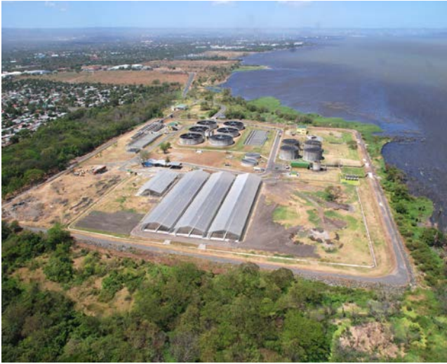
The new treatment plant is again making Managua an attractive body of water on the capital's doorstep. Source: KfW
