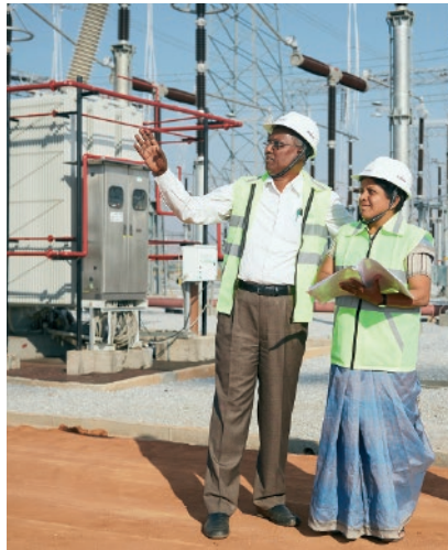
Transmission lines and substations feed sustainably generated electricity into the Indian power grid to transport it to where it is needed most.
