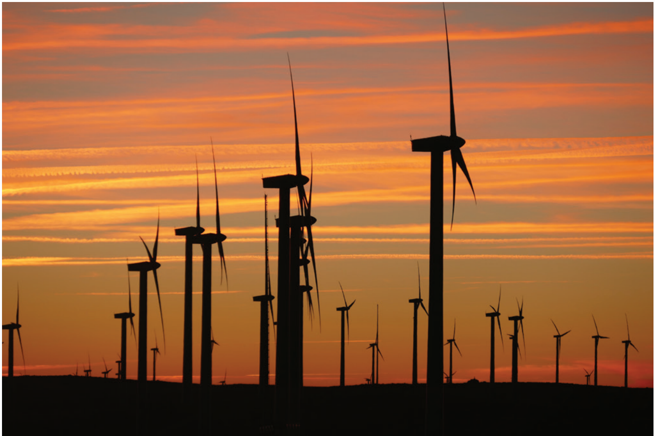
Wind Energy Facility, Valencia region, Spain. Photo: Alvaro Camiña
