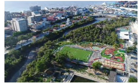
Beira/Mozambique: Thanks to a combination of green and structural infrastructure, the city of Beira in Mozambique now has effective flood control. KfW/TPF
