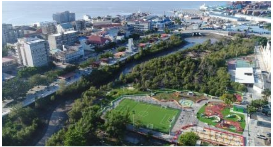
Thanks to a combination of green and structural infrastructure, the city of Beira in Mozambique now has effective flood control. KfW/TPF
