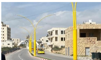
Street restoration and lighting at an entrance to the town of Jannatah. Source: KfW / Hannah Linnemann
