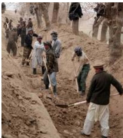
Road construction in Afghanistan
