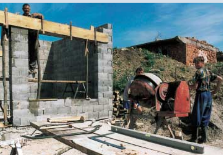
Rebuilding a destroyed home.
