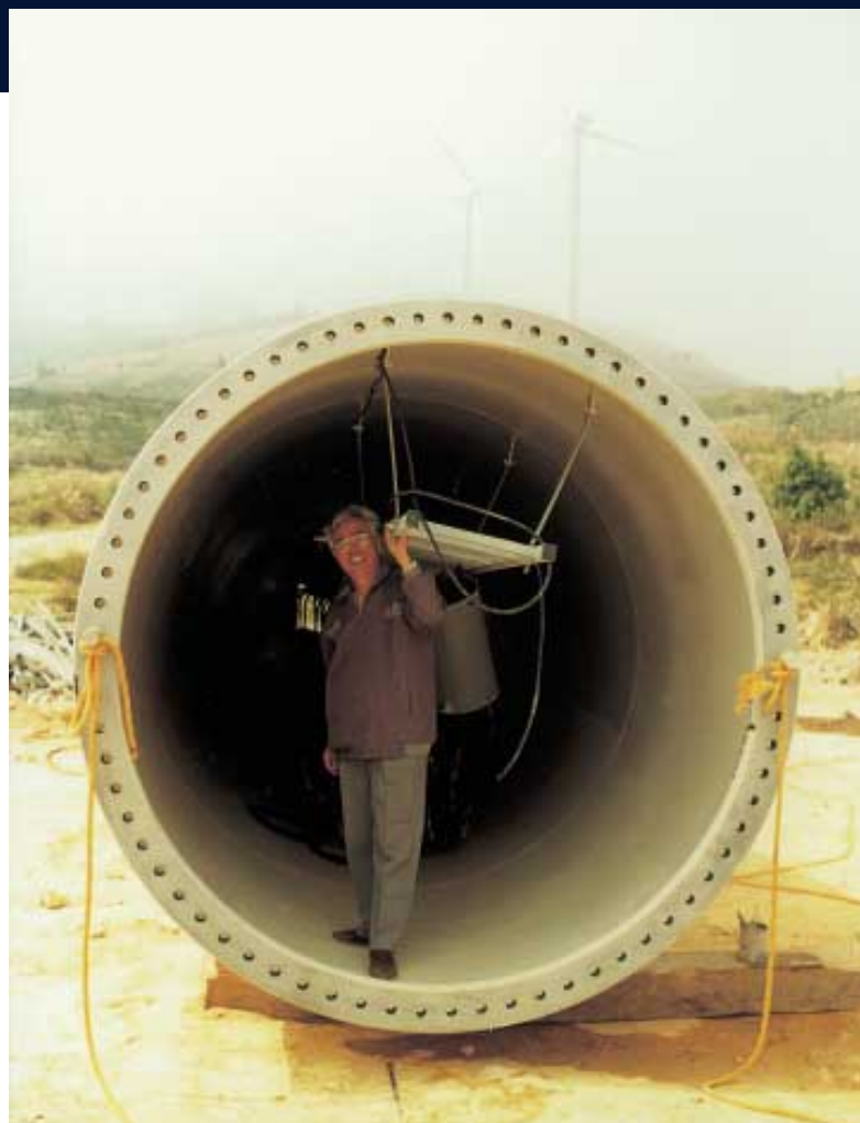
Innovations that shape the future: promoting renewable energy – wind park in China.
