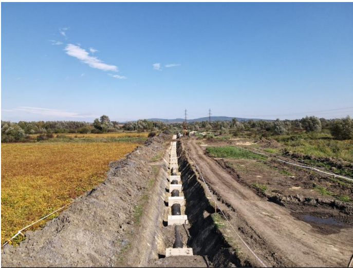
A water pipe is being rehabilitated in Chernivtsi. Source: Hennadii Dudko, Head of Strategic Development Department Chernivtsivodokanal
