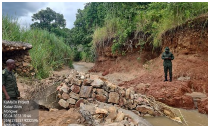
Irrigation works in Magatianthi district. Source: AHT Group GmbH, Bhundia Associates; AHT Group
