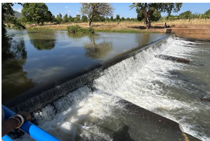
Inlet structure in Kiramanti. Source: KfW, 2025 Dirk Wenzel
