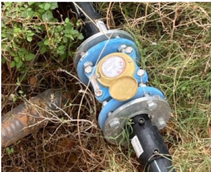
Modernised drinking water access for rural households. Source: KfW / Daniela Casabona-Fischer
