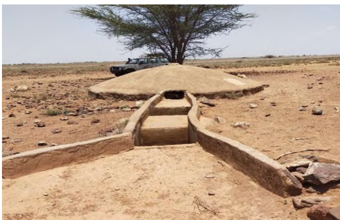
Underground water tank to extract surface water during the rainy season at Kubi Adhi. Source: GOPA
