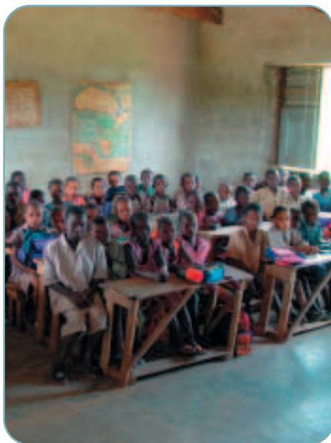
Classroom before rehabilitation.
